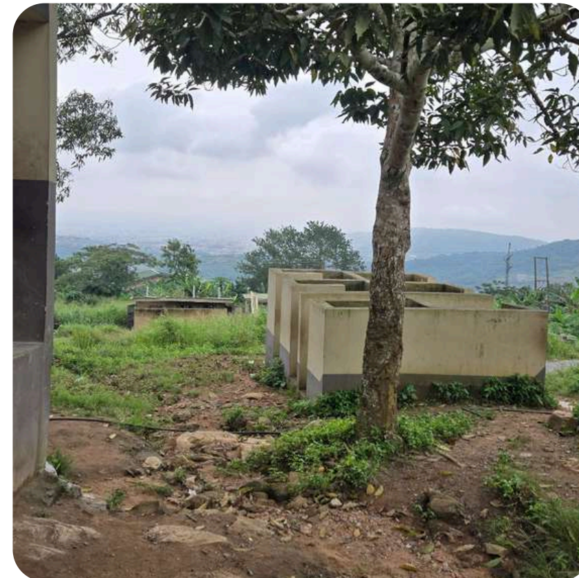
2026 Project - Building a new washroom
